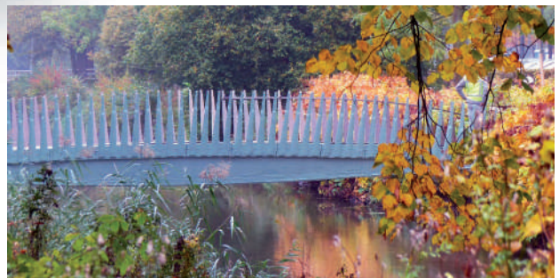
FIG. 36 A 14-meter-long bridge made from flax & hemp fiber composites in Eindhoven, The Netherlands. The bridge was built as part of a research project by the Technical University of Eindhoven. (TU Eindhoven)
