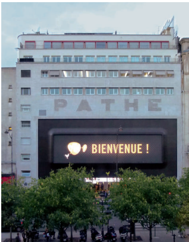
FIG. 21 Large facade panel encapsulating a screen mounted above the entrance of a local movie theater in Paris. The panel is reinforced by a flax fiber weave. (Woven flax fabric /Groupe Depestele used by Pathé Cinema in Paris, France and produced by Multiplast).
