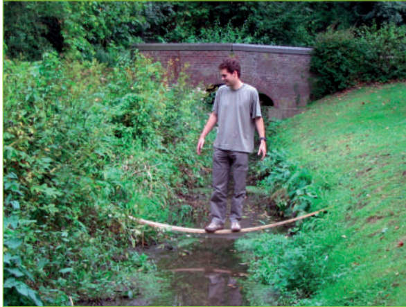
Figure 3: A wooden beam over a brook: not very stiff, but sufficiently strong to withstand the weight of one person.
